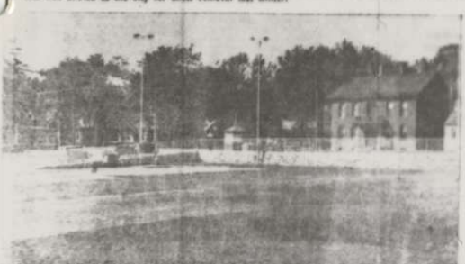
Lafayette square between Fourth and Fifth and Adams and Brown street has been improved by removal of trees, curbing on the north side, installation of 500 feet of chain mesh fence, five feet in, repair of the cement station, construction of a concrete wall around the walking post and of a concrete sidewalk diamond shape. Expenditures total $7,200 including snow removal allowances.
