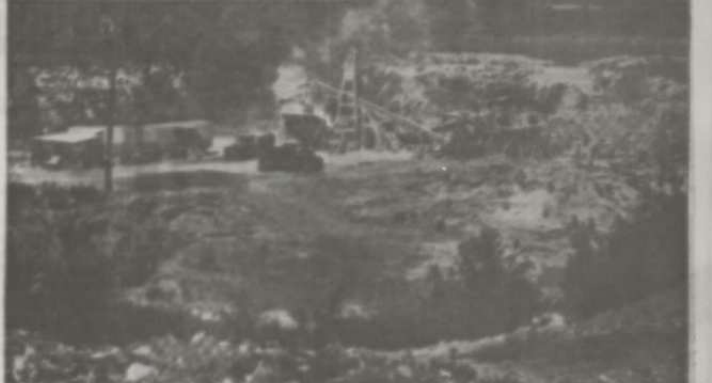
Source of crushed stone and sand for improvement of county roads, city streets and drives and park drives, is the county quarry at Greenport. Material placed in application. Expenditures have been $20,000, mostly for wages, part allocated to snow removal and streets. A survey of building has passed out for improving drive in that town. Federal expenditures have totaled $20,000.
