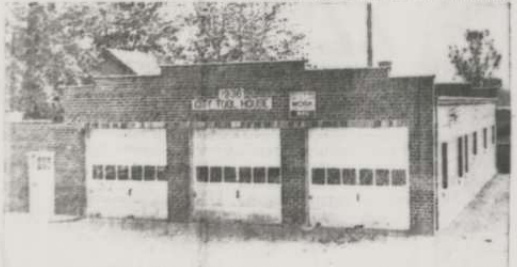
Greenport now has a neat appearing, substantial brick and concrete tool house and garage. Important feature is complete machinery owned by the city thru the aid of WPA funds. Expenditures of federal funds amounted to $7,300, but part of this was used to remove snow from streets and sidewalks in 1935.
