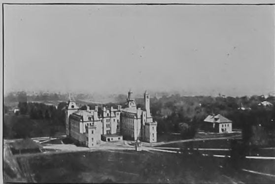
REAR OF OLD MAIN
