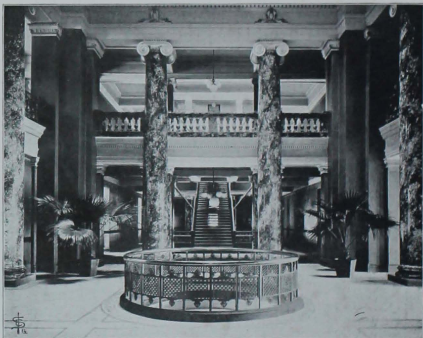
INSIDE OF NEW MAIN
