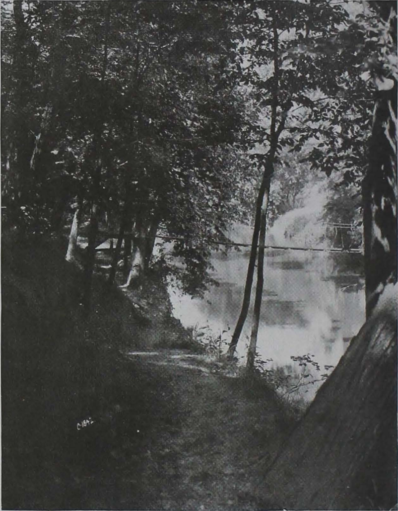
BRIDGE OVER SQUAW CREEK
