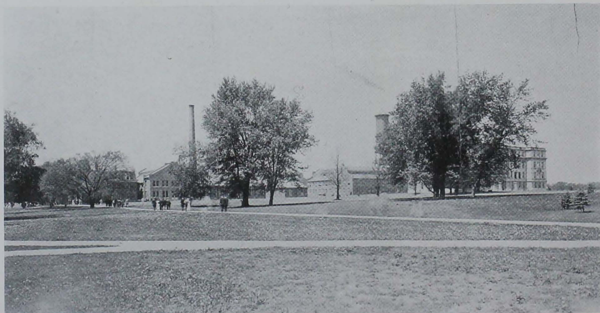
GENERAL VIEW OF ENGINEERING BUILDINGS
