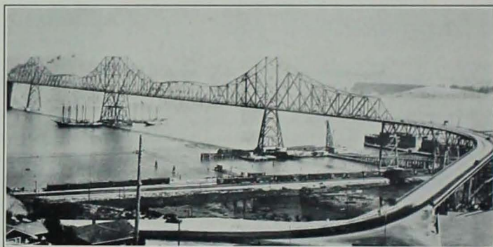
Steel Highway Bridges
