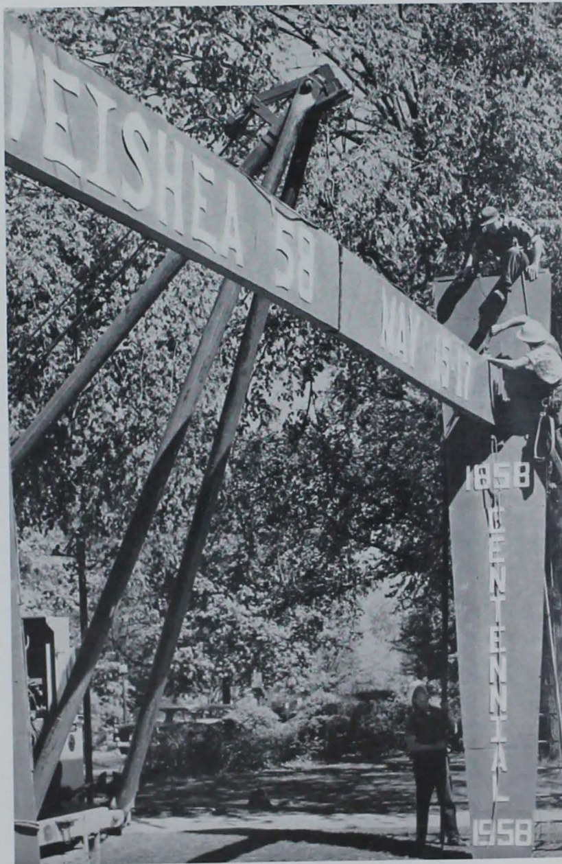
WORKMEN ERECT the giant banner spanning Lincoln Way to welcome visitors to 1958 Veishea, this year's event denoting the celebration of Iowa State's centennial.
