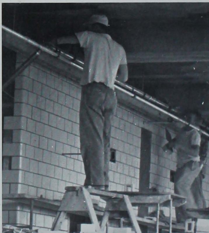
During the winter months construction on the interior of the new Science Building advanced rapidly.
