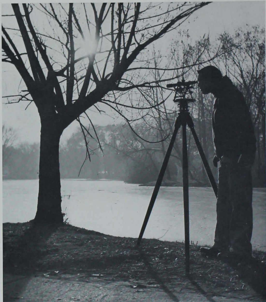
Engineer brings view of Union into sights
