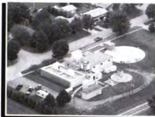
Charles City Water Plant upgrades and expansions
