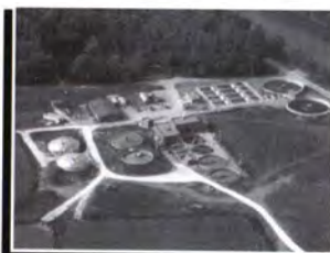
Improving water quality on the Des Moines River - Fort Dodge Wastewater Treatment Plant improvements
