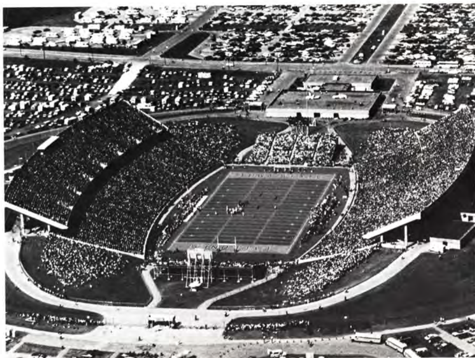
Cyclone Stadium-Jack Trice Field
