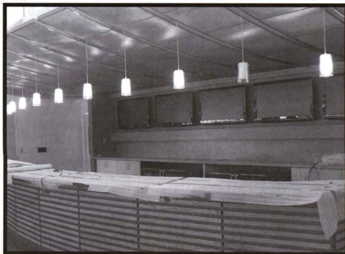
The Jack Trice Club is located in the east concourse of Jack Trice Stadium. A total of 572 seats have been added to the club section. Here is a view of the bar area.
