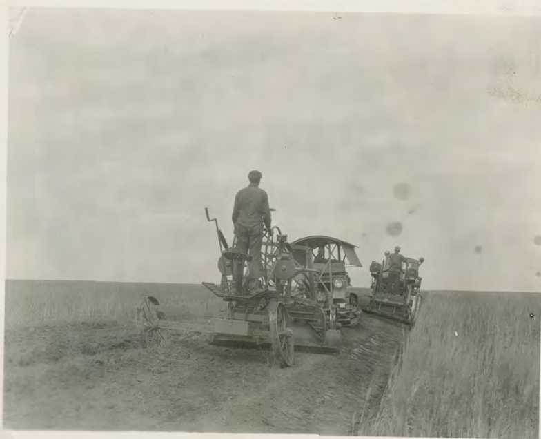
Making roads. Sewky No. 2
