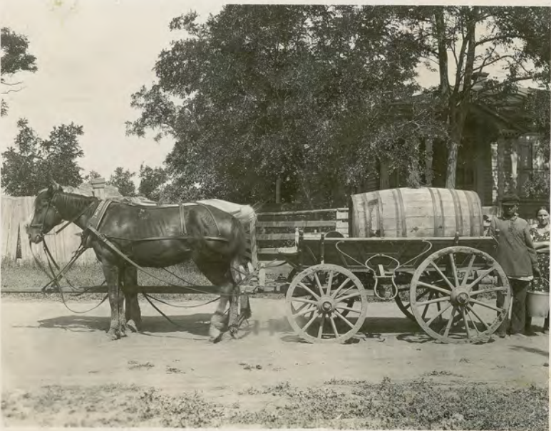
The village water system
