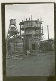
Constructing our water tower
