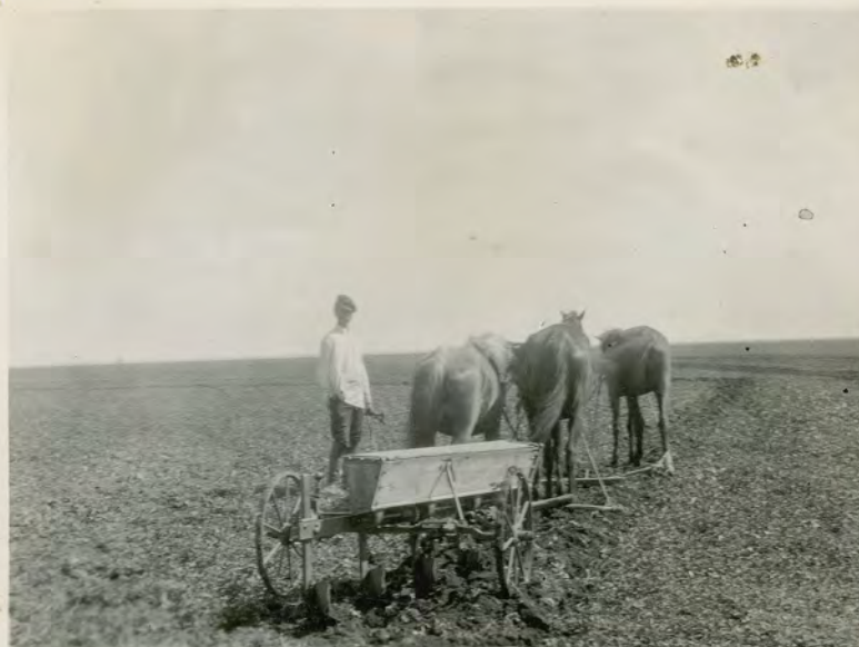
The principal type of peasant drill implement use in Ukraine - called a "Booker" Drills the grain and little 6" flows cover it
