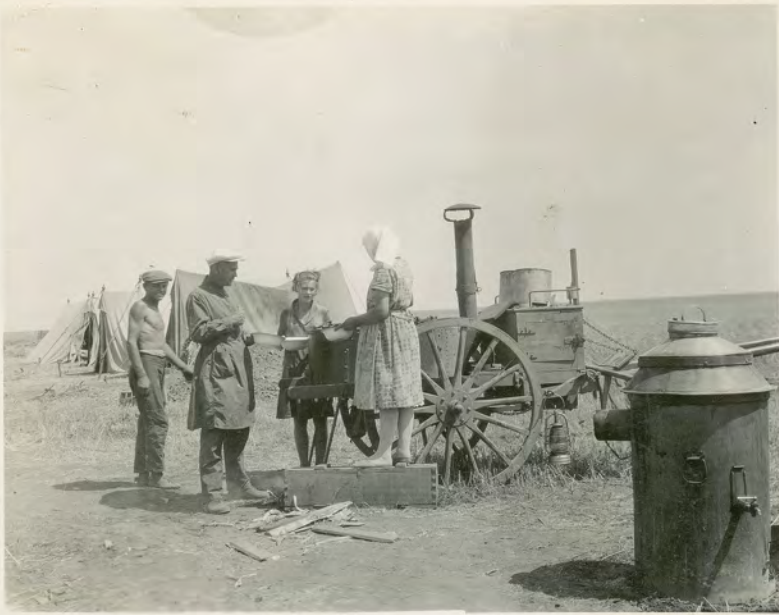
Field camp soup kettle and water boiler
