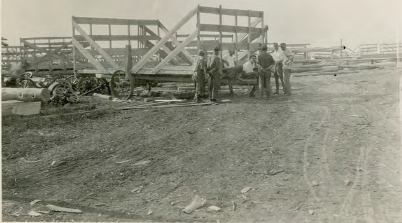
Bundle wagons to be used on the giant Sorkhoz. Made to hold 2 1/2 acres and be pulled by an D.H.C. 10-20. Designed by a Russian Engineer was a failure
