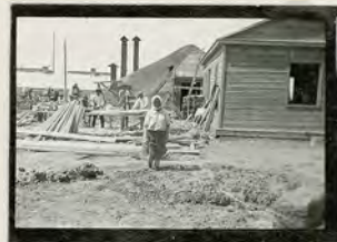
Making mud plaster by foot (feet) Used for exterior and interior
