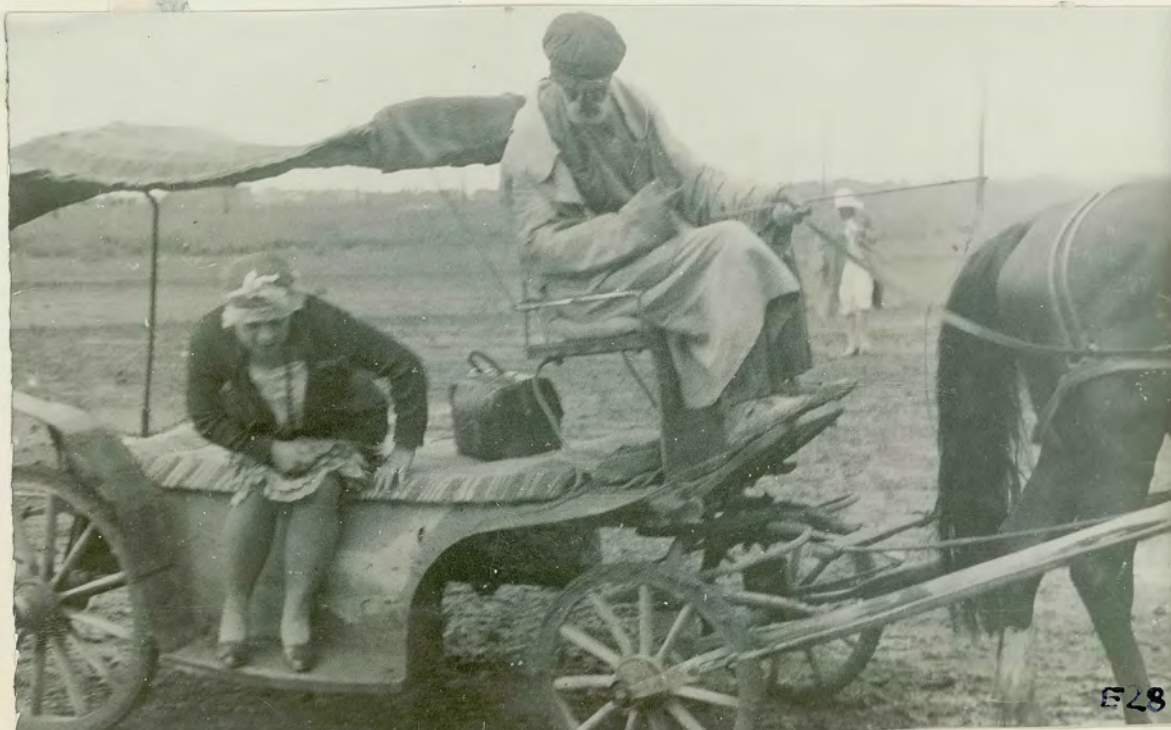
CLOSE INSPECTION OF THE ROAD
