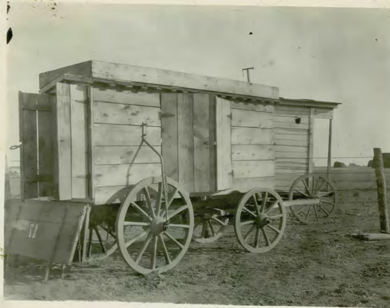
Field blacksmith shop
