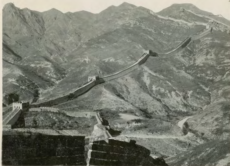
The Great Wall at Nankow Pass
