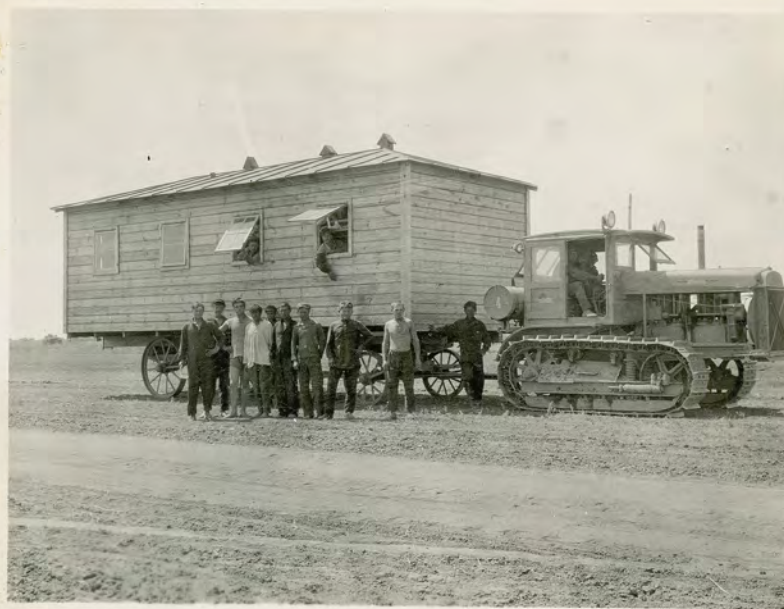
Above: Night shift morning camp, Sukhoi No. 2. Aug 24 neg # 0068800
