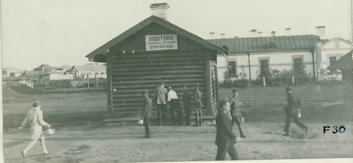
A HOT WATER TANK IN UKRAINE
