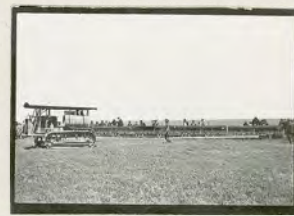
Stirny demonstrates a cable hitch on a 70ft drill spread
