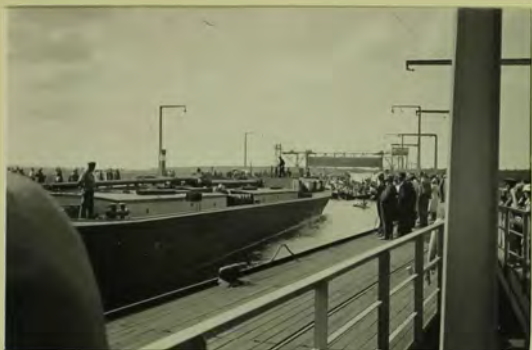
SHIP LIFT - Upperside - Elbe Northeast of Berlin
