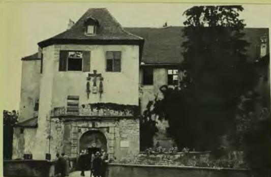
BRIDGE AT MEERSBURG CASTLE
