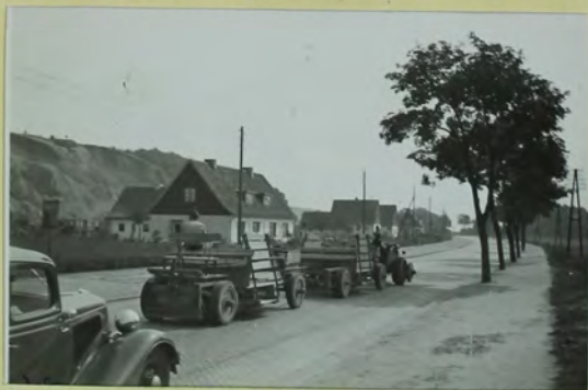
ROAD OUTFIT Pulled by Lantz Bulldog tractor D28
