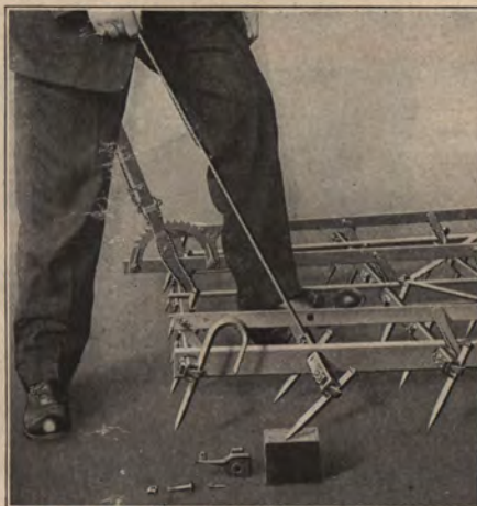
Showing what will happen to a harrow not equipped with strengthening bar under same conditions Note that the pressure of only one foot will cause sagging
