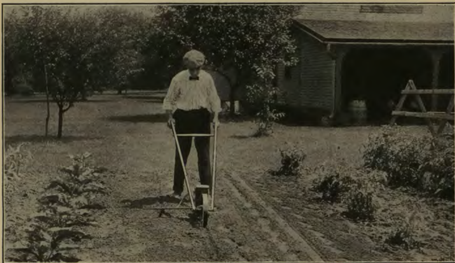
Planet Jr. No. 4 Seeder opening the furrow, planting the seed, covering, rolling down and marking out the next row, all in one operation
