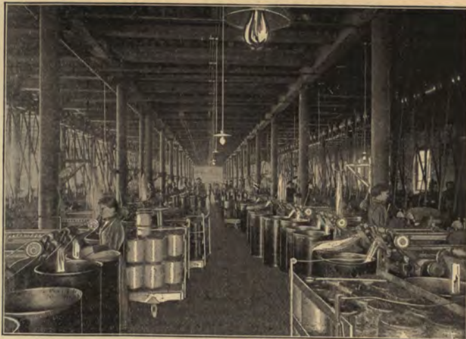
Row of Finishers in Mill No. 2.
