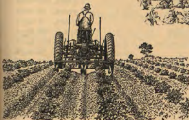
Right: John Deere Two-Row Cultivators for listed crops. Hydraulic power lift.
