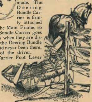
THE DEERING BUNDLE CARRIER. Its fingers fold when they strike an obstruction.
