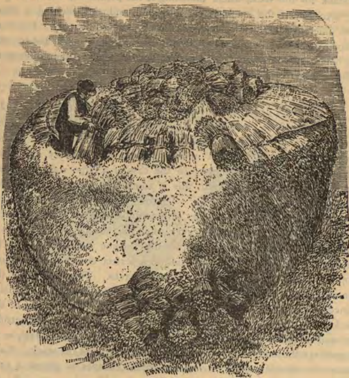
The Stack as carried up from the ground.
