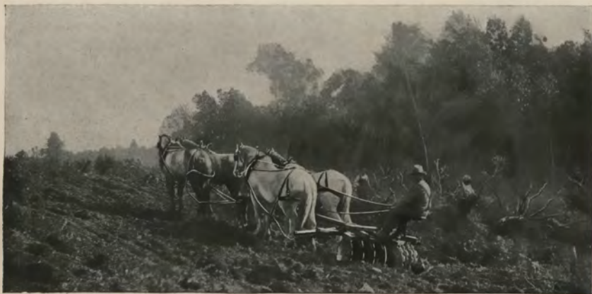
The Bush and Bog Plow at work after dynamite and fire had done their work
