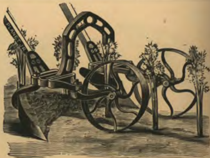
Fig. 15—The "Planet Jr." Double-Wheel Hoe, earthing up.
