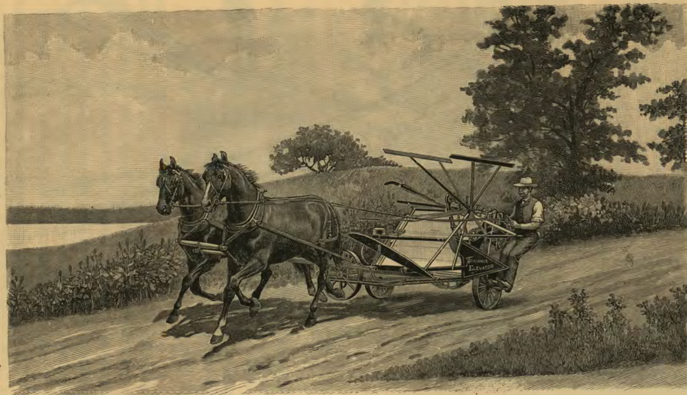
ADRIANCE ELEVATOR BINDER ON TRANSPORT.
