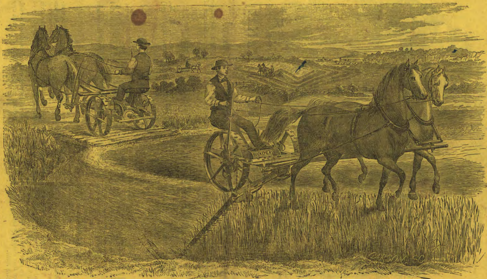
Cutting out a Ditch.
