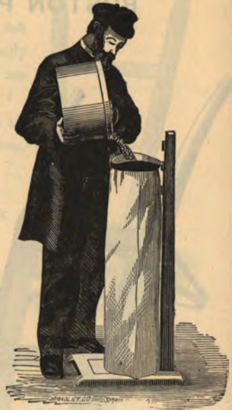
THE NEW WAY.
