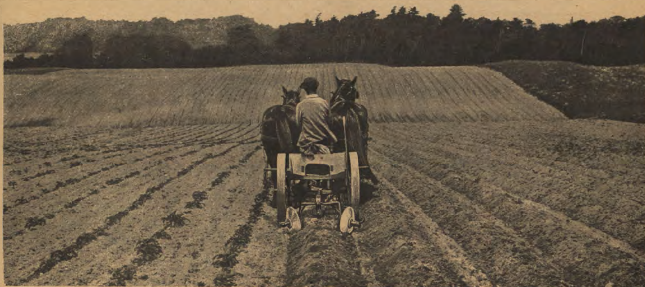
"IRON AGE" (Improved Robbins) Planter making second application of fertilizer, covering it and ridging the potatoes at the same time
