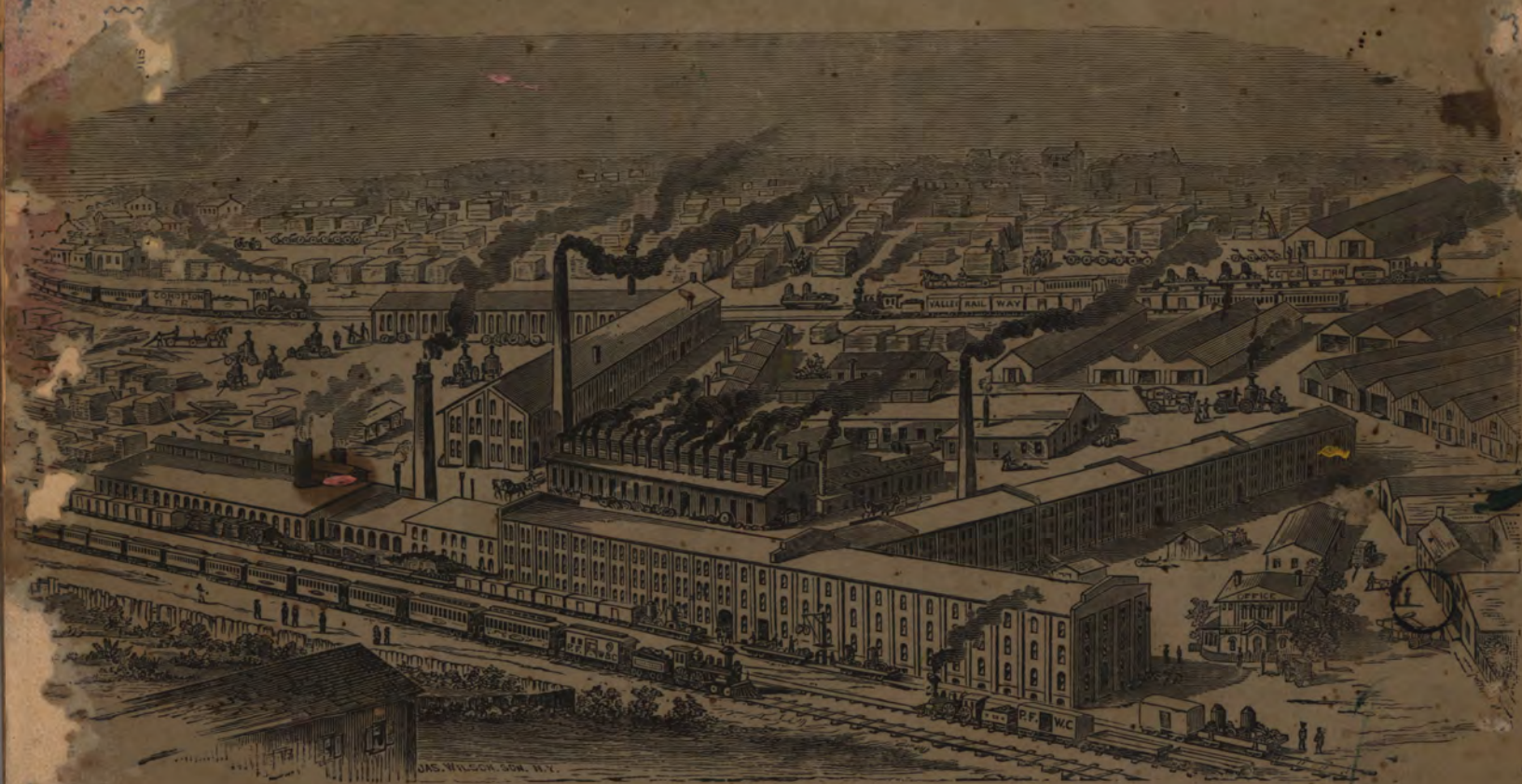
C. AULTMAN & CO'S WORKS AT CANTON, OHIO.
