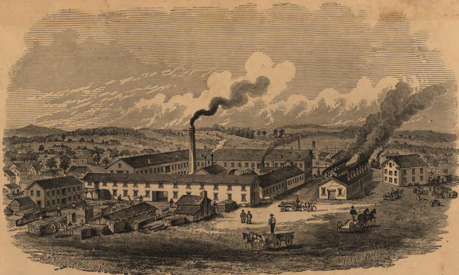
REAR VIEW OF WORKS.
