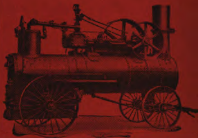
Farquhar Locomotive Rig
