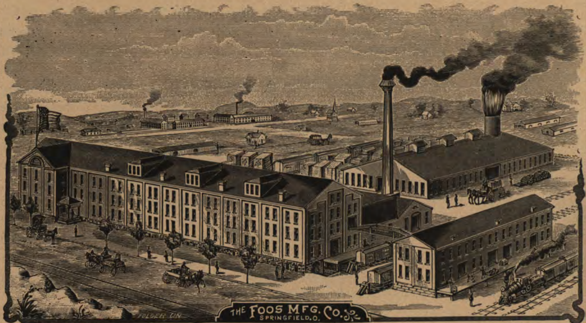
NEW WORKS ERECTED 1890.—Dimensions: Main Building, 60 x 230 Feet, Four Floors and Basement. Blacksmith Shop, 24 x 34 Feet. Warehouse 50 x 125. Foundry, 80 x 150 Feet.
