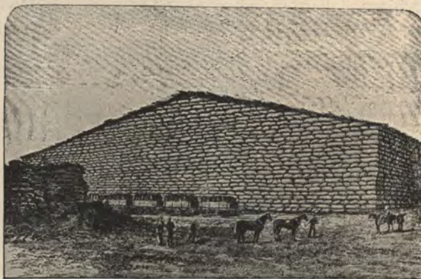
This stack of 35,000 wheat sacks was erected by a grain buying firm at Caltowie, South Australia. Storage facilities in that country are limited, and the plan shown in our illustration is in common use.
