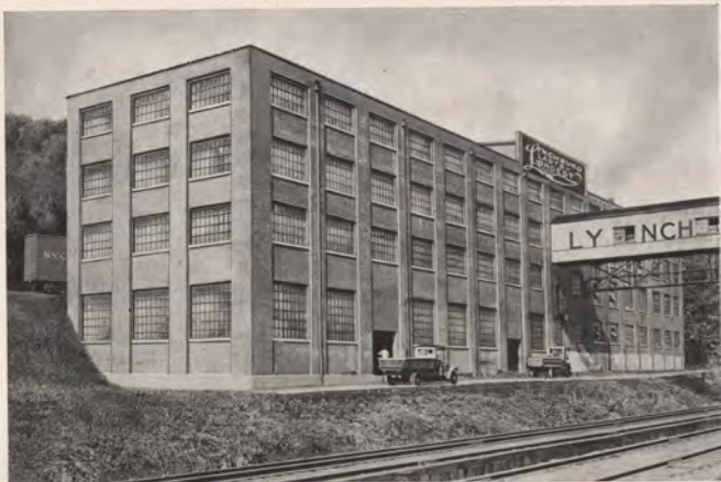
FIRE-PROOF WAREHOUSE, STORAGE CAPACITY OF 300 CARLOADS OF PLOWS AND PARTS
