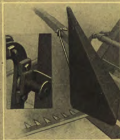
Platform, Connections—Front and Rear and Roller Box. Finger Bar Stiffener. Torsion Pipe. Pole and Frame Connections. Grain Wheel and Folding Dividers.
