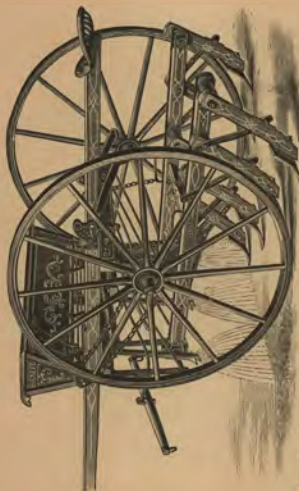
New Senior Buckeye Cultivator with Wood Beams, Wood Standards and Seeding Attachment.
