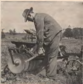
It takes but a few moments to apply the transport trucks, which are a great protection to the disks when traveling over stony roads
