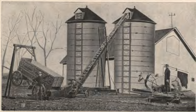
An Everlasting Sandwich Cypress Farm Elevator Used as a Silo Filler
