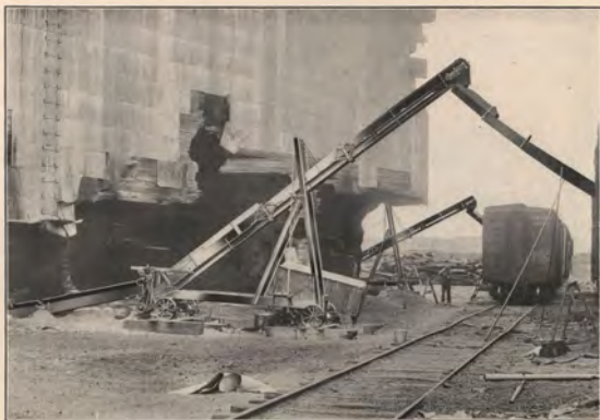
Two Sandwich Farm Elevators Installed at the Ruins of The Iowa Elevator Co., Peoria, Illinois, which was Recently Destroyed by Fire
