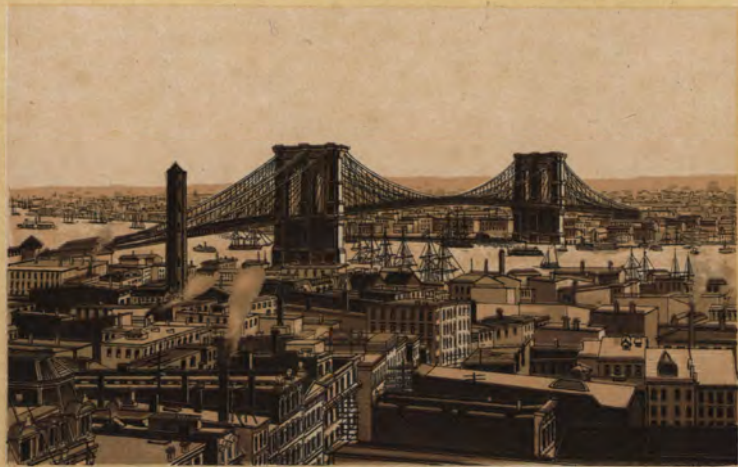
EAST RIVER BRIDGE.
