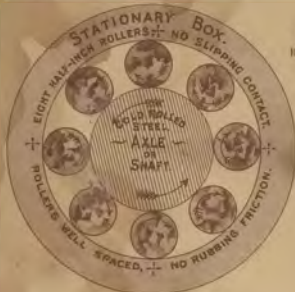
ANTI-FRICTION BEARING.
