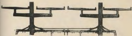
Four-Horse Chain Equalizer Hitch, Two Poles.
