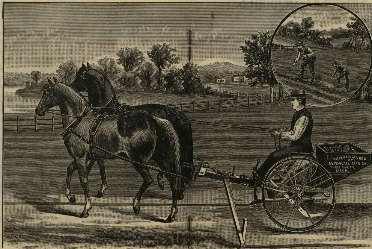
The Aspinwall Potato Planter at work in the field, doing the Entire Work of Marking, Furrowing, Dropping and Covering, all in One Operation.
