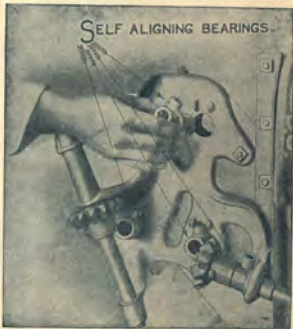
Self-aligning Bearings and Removable Boxes prevent Cramping or Binding and Insure Light Draft.
