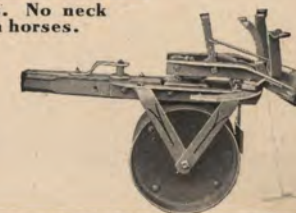
View No. 7. Rigid front wheel. Has a lock to hold wheel in center.
