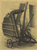
Reaper Gearing. Roller Bearings. Grain Wheel and Outer Divider. Raising Lever and Suspending Bar. Rake parallel with Bar. Automatic Trip. Rake Standard. Platform Support and Braces. Reaper Folded.
