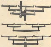
Showing special Hitch for three horses with Set-over Pole, and special 4-horse Hitch and 3-horse Hitch for Tongue Truck.
