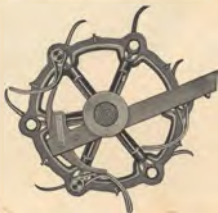
Sectional view of gathering drum.
