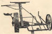
Showing Frame, large Main Wheel, location of Pole and Seat.
