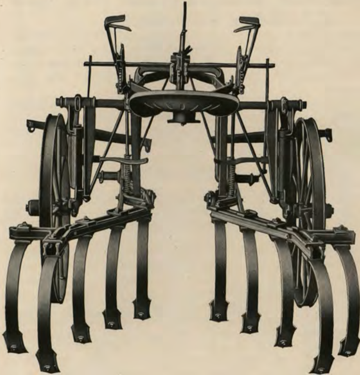
Rear View No. 208 Buckeye Narrow Row Pivot Axle Riding Cultivator
