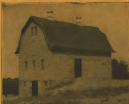
Dairy Barn on the Hudson Farm
