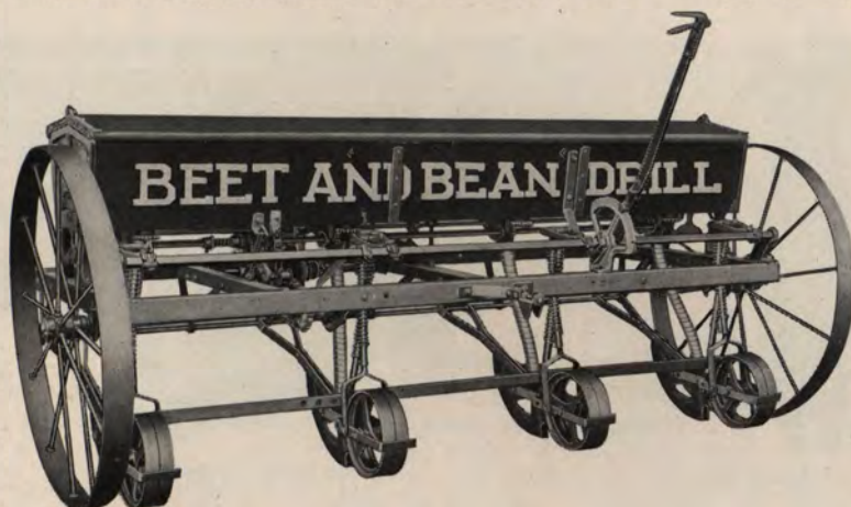
The Superior No. 7 Four-Row Shoe Beet and Bean Drill, Fertilizer Style.
